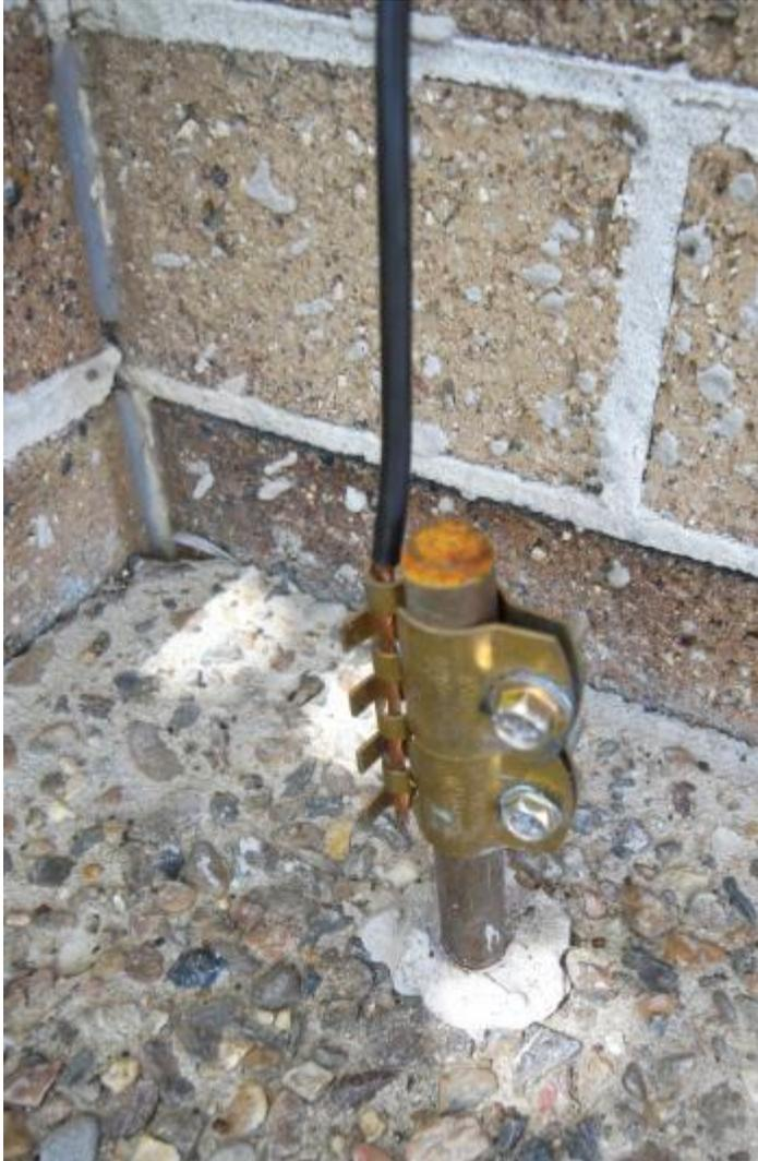
Lastly, earthing strap connected to the body of the cabinet, and leading outside to an 8 foot copper earth spike driven into the ground (drive into earth under concrete because the ground is more moist for better earthing beneath concrete).
